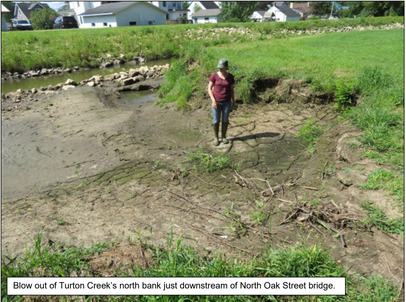
High flows overtopped the berm along Turton Creek and eroded the back side of the berm as can be seen here. See 2017 aerials that show extensive alluvial fan spreading out into wetlands to the north.
